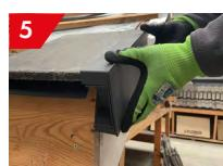
5 Fit the first verge section making sure that it is located firmly onto the eaves starter. Once in position the verge unit can be screw fixed into the end of the batten using 40 x 3.5mm stainless steel screws.
