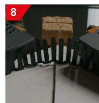
8 When we reach the top or apex of the roof, we can close this area off by using the ridge comb that is supplied as part of the eave and ridge kit. The teeth of the comb sit over the bottom edge of the verge unit where it will be held in place. If using a dry ridge system the ridge roll can be extended over and tucked back up underneath to offer additional protection.
