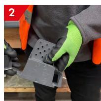
2 The eaves starter piece, which is part of the eave and ridge pack, should be used to fix the first verge unit. This will first need to be cut as marked to suit either the left or right hand verge.
