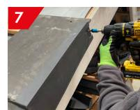
7 This process can now be repeated, ensuring each verge unit engages with the one below, so a verge unit covers the end of every course of tiles and all are securely fixed into the batten end. Ensure the small 3mm gap is maintained on every course.
