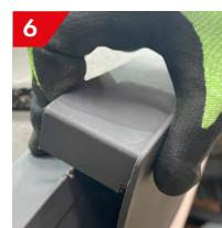
6 The second verge can now be positioned by locating the front edge of the verge over the notched section of the installed verge, and sliding up until it meets the leading edge of the tile. If there is a significant change of pitch between the eaves and second course it may be easier to put the verge in position first and slide the tile into it. Then fix to batten end.
