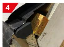
4 An additional batten behind the fascia board can also be used if required to ensure a suitable fixing point - this should be securely fixed to the rafters.
