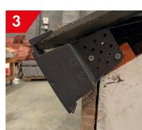
3 Place the eaves starter in position, flat on top of the tile and twice fix into the end of the fascia board, brickwork or timber tilt fillet. On the left hand verge the side interlock of the tile should be removed on all verge tiles.
