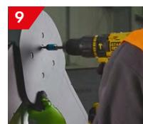
9 To finish screw fix the Ridge End Cap to the ridge batten, securing it in place and completing the Ambi Verge system. The ridge system will need to be installed prior to fixing this. If required a small slot can easily be made on each side of the end cap so it sits over the upstand of the verge unit.
