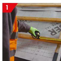
1 Extend the tiling batten. Once the roof has been felted, you will need to install the tiling battens, ensuring they are extended 38mm beyond the gable wall, barge board or render. This will allow for screw fixing of the verge.
